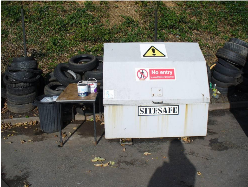
Figure 17 Improperly Stored Waste
