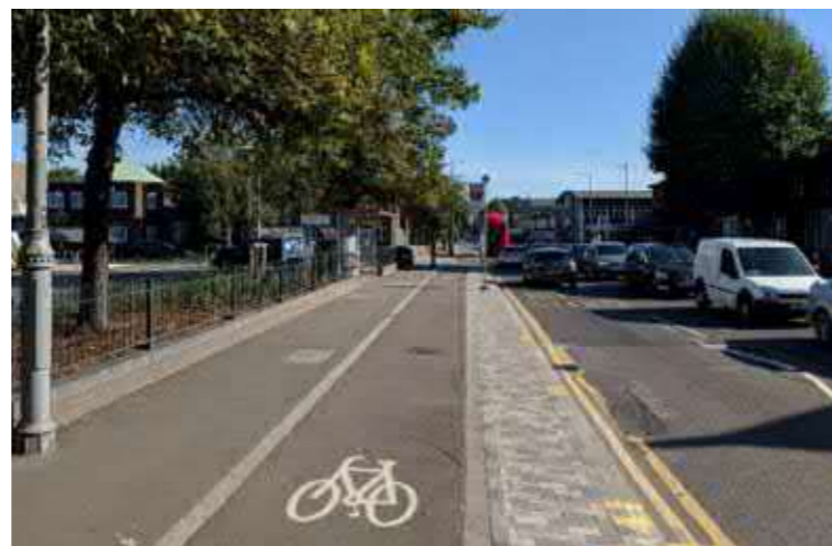
Figure 3.8. Stepped cycle track (intermediate height)
