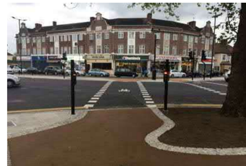
Figure 4.8. Improved signalised junction (Enfield)
