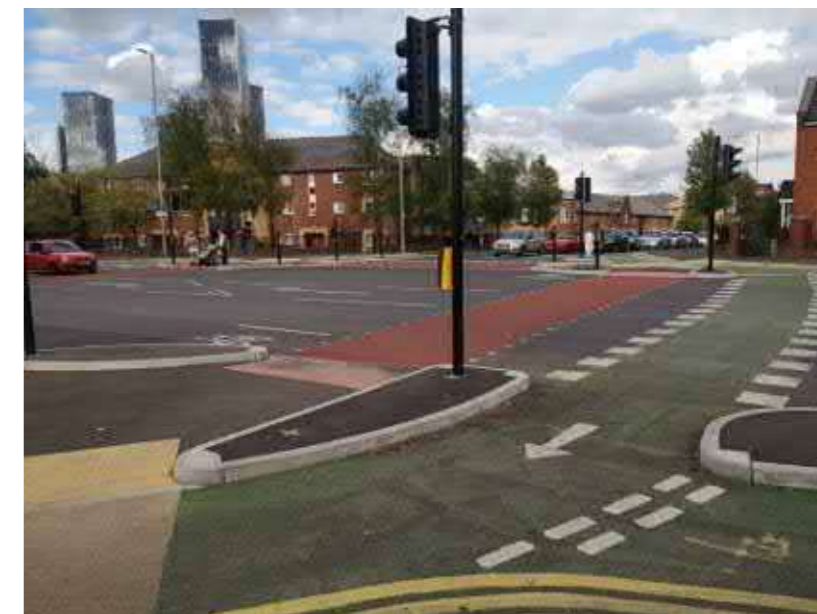
Figure 3.12. CYCLOPS signalised junction
