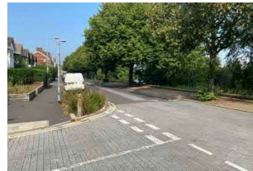
Figure 4.7. Buildouts with SUDs
