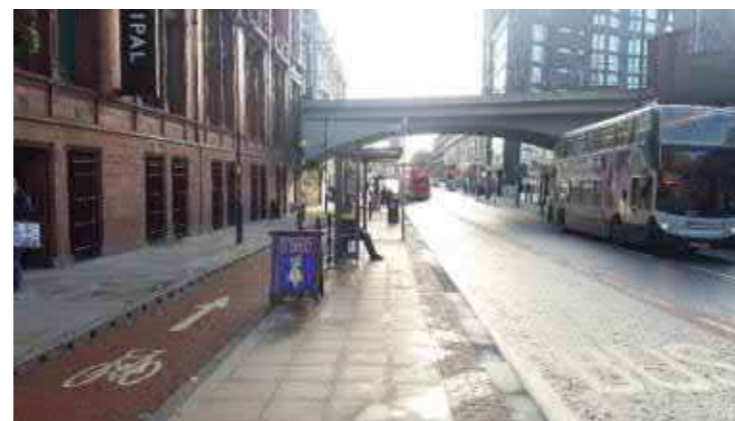
Figure 3.7. Segregated cycleway (carriageway height)
