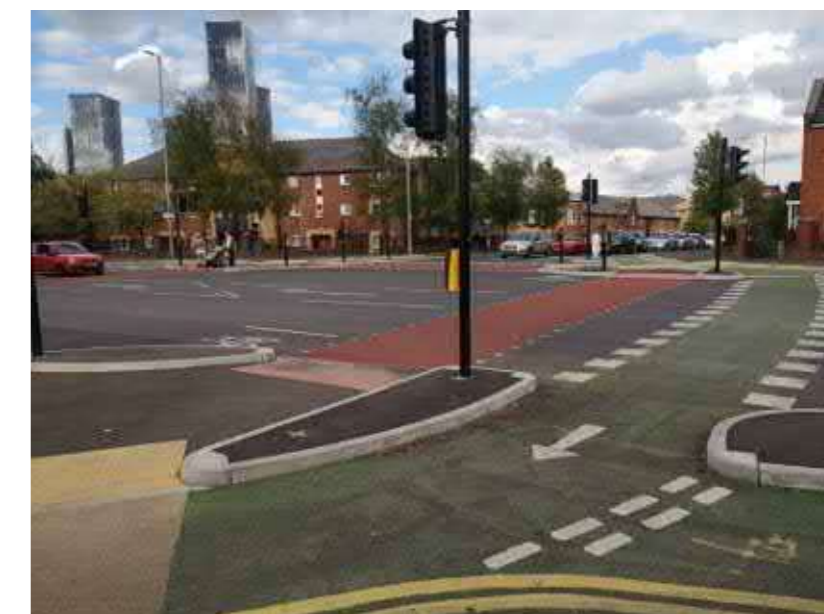
Figure 3.12. CYCLOPS signalised junction
