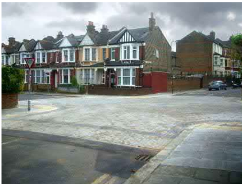
Figure 4.9. Raised table junction
