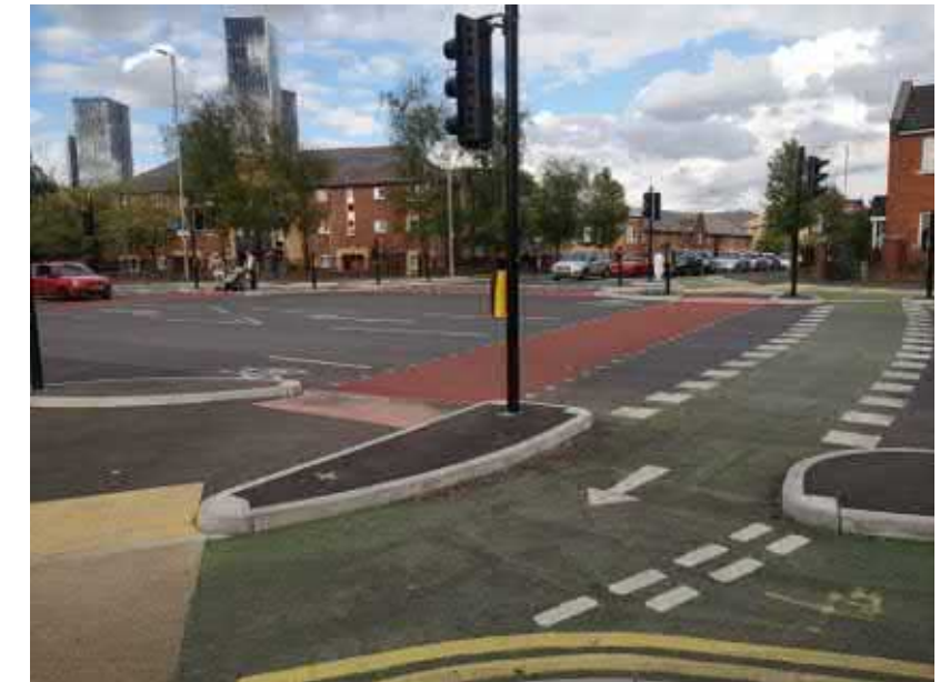
Figure 3.12. CYCLOPS signalised junction
