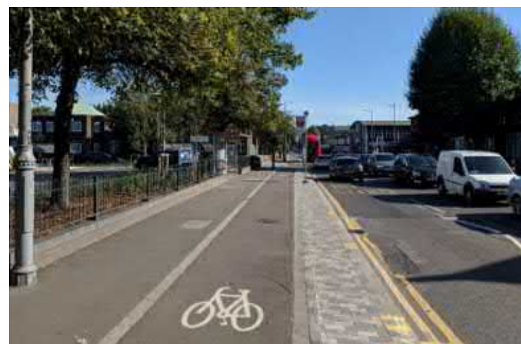
Figure 3.8. Stepped cycle track (intermediate height)
