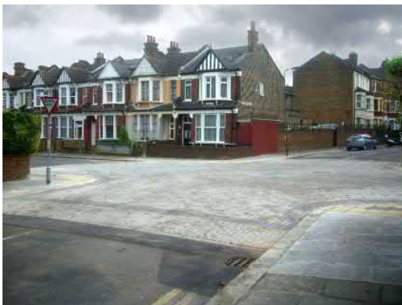
Figure 4.9. Raised table junction
