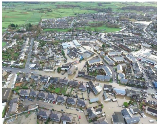
Figure 2: Impact of Storm Desmond flooding at the A685 and across Kendal
