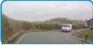
Passing point and retaining wall
